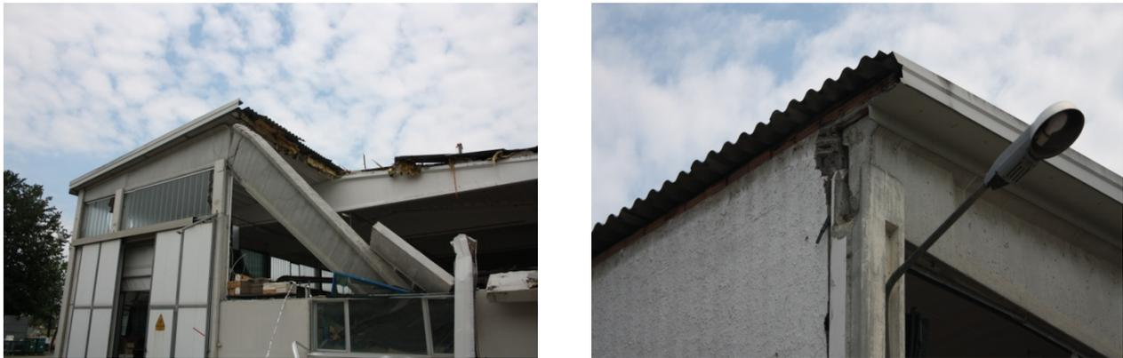
**Figure 1.1 Failure due to loss of support of the beam during the May 2012 Emilia-Romagna earthquake in Northern Italy [Belleri et al. [1]].**
