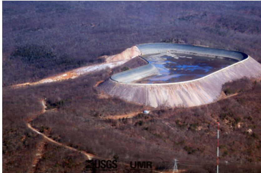
Fig. 3.1 Aerial view of the Taum Sauk dam following its overtopping and failure, in 2005. U.S. Geological Survey.
