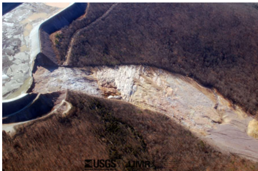
Fig. 3.2 Aerial view of part of the area affected by the Taum Sauk dam-break wave. U.S. Geological Survey.
