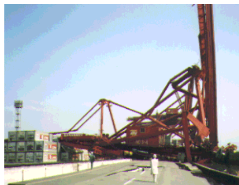
Fig. 6.8 Crane total collapse. Various damages to other cranes like plastic hinges and bending of their members (Rokko Island)
