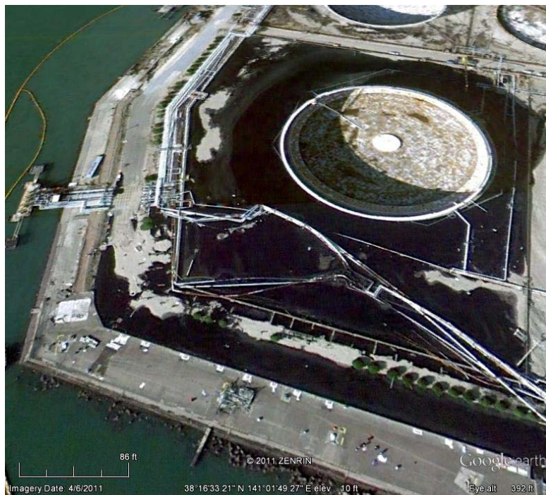
Fig. 2.12 Heavy oil release due to tsunami-triggered damage at the Sendai refinery (©2011 Google, ZENRIN)
