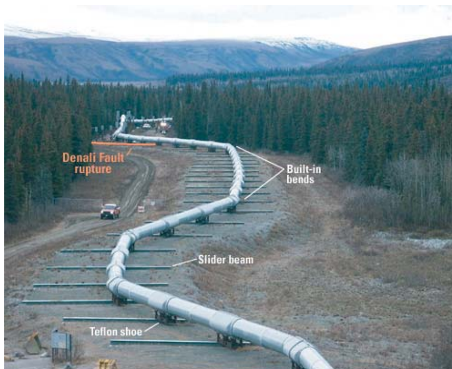
Fig. 4.3 Trans-Alaska pipeline crossing the Denali fault line (USGS, 2003)
