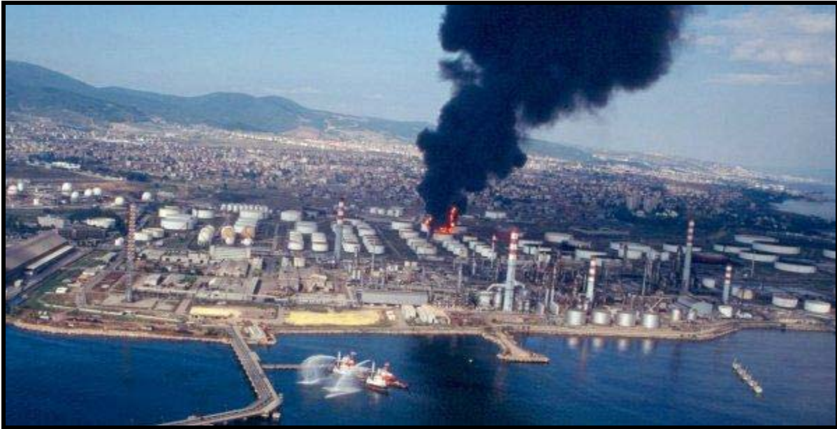
Fig. 2.3 Aerial view of the Tupras refinery after the Kocaeli earthquake
