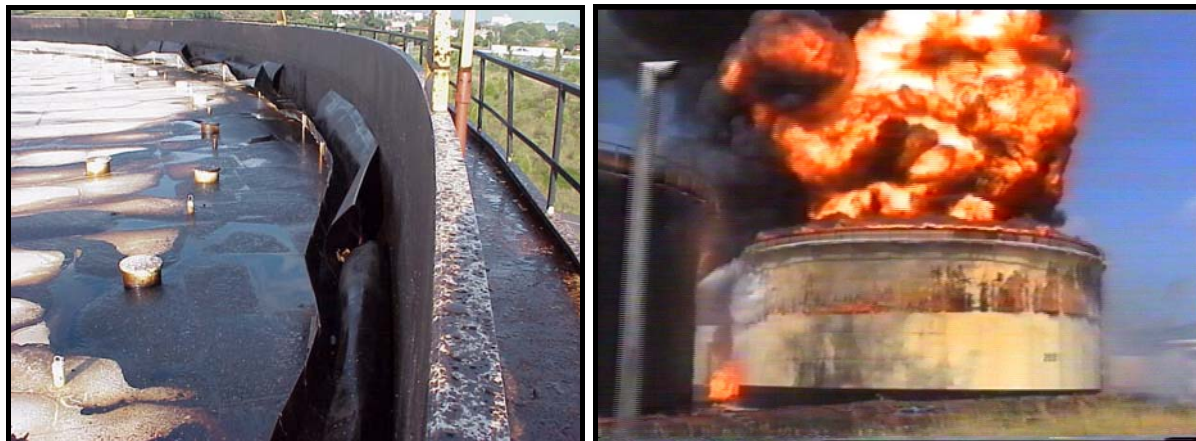
Fig. 2.4 Tank fire at Tupras refinery due to collision of the floating roof with the tank wall (Courtesy of Tupras A.Ş. (TUPRAS, 2000))
