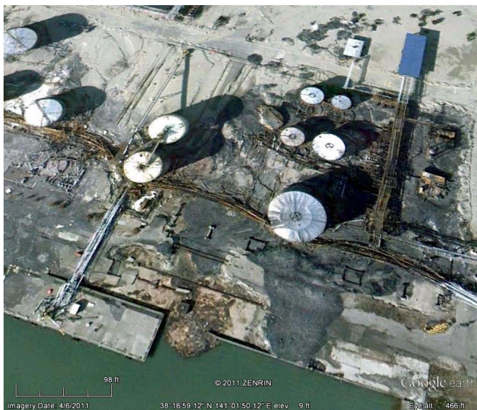
Fig. 2.10 Part of the Sendai refinery's western section that was consumed by flames (©2011 Google, ZENRIN)
