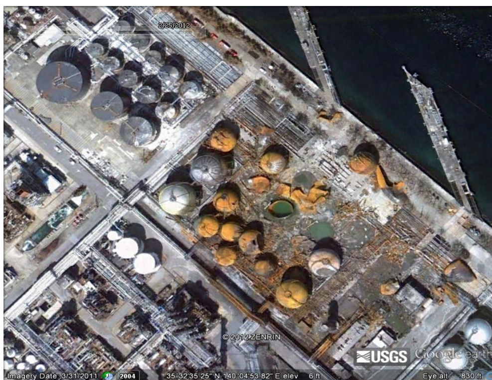
Fig. 2.1 The LPG tank farm at the Chiba refinery after the earthquake-triggered fires and explosions (©2012 Google, ZENRIN)
