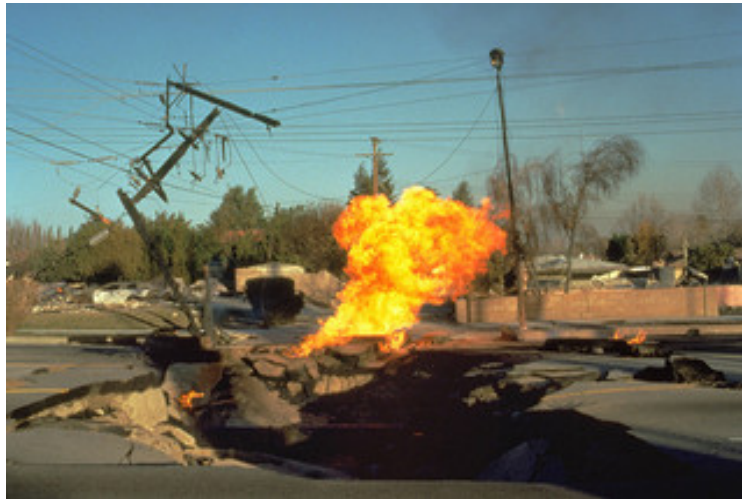
Fig. 5.12 Burning of leaked gas from ruptured gas line
