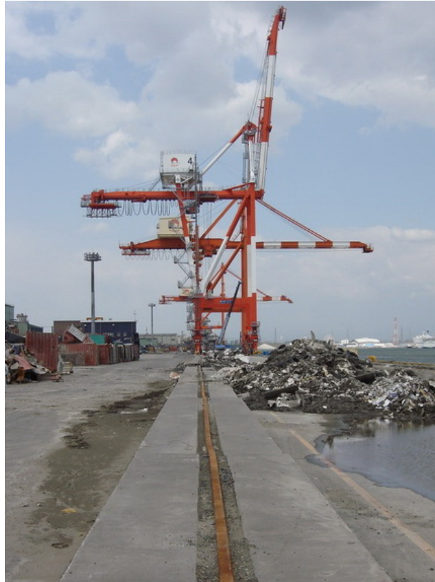
Fig. 6.20 Landside crane rails at the eastern side of Takasago Wharf (Percher, 2014)
